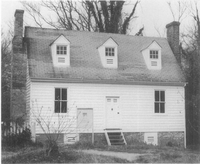
Figure 10. Regrading around the Booker Tenement at Colonial Williamsburg has protected the masonry foundation wall from excessive damp. This building has been successfully mothballed for over 10 years. Note the attic and basement vents, the temporary stairs, and the informative sign interpreting the history of this building.
