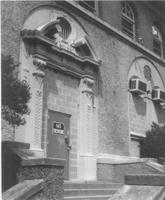
Figure 12. First floor openings have been filled with cinderblocks and doors, window sash and frames have been removed for safe keeping. Note the security light over the windows and the use of a security metal door with heavy duty locks. Photo: H. Ward Jandl, NPS.
