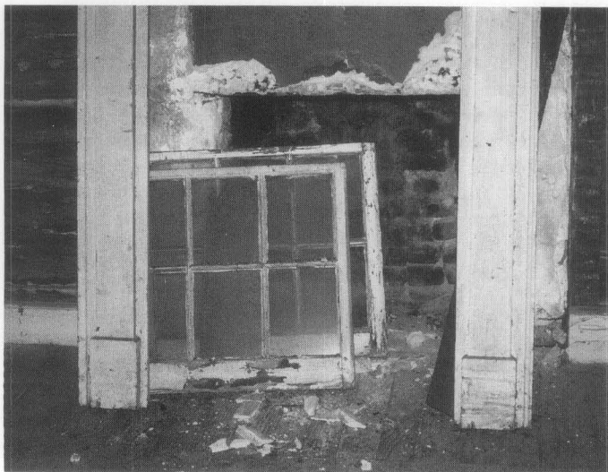
Figure 5. Loose or detached elements should be identified, tagged and stored, preferably on site. Photo: NPS files.
