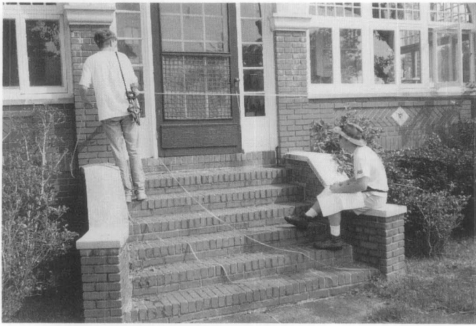
Figure 4. Documenting the building's history, preparing schematic plans, and assessing the condition of the building will provide necessary information on which to set priorities for stabilization and repair prior to securing the building. Photo: Frederick Lindstrom, HABS.
