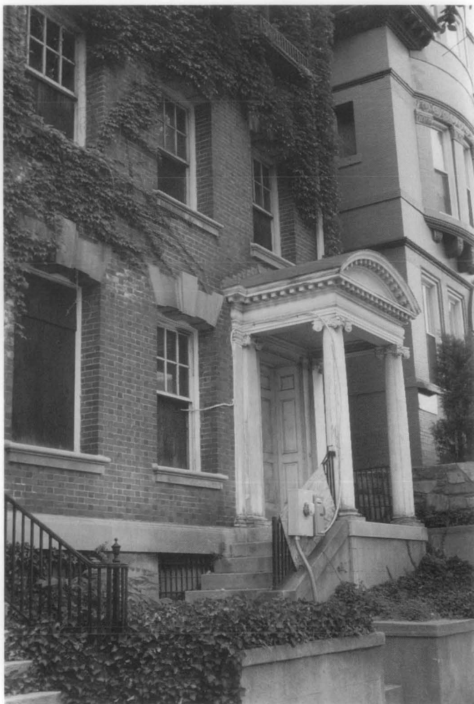
Figure 22. All systems except temporary electric have been shut off at this residence which has been mothballed over 20 years. An electric meter and 100 amp panel box have been set on a plywood panel at the front of the building. It is used for interior lighting and various alarm systems. The building, however, is showing signs of moisture problems with efflorescent stains on the masonry indicating the need for gutter maintenance and additional ventilation for the interior. The vegetation on the walls, although picturesque, traps moisture and is damaging to the masonry. Photo: H. Ward Jandl, NPS.
