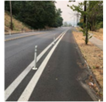
Physically Separated Bike Lane
