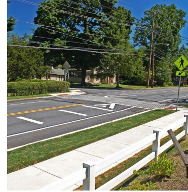
Raised Crosswalk/ Intersection
